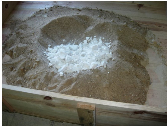
Figure 4 - Introduction of the quicklime into the sand mix
